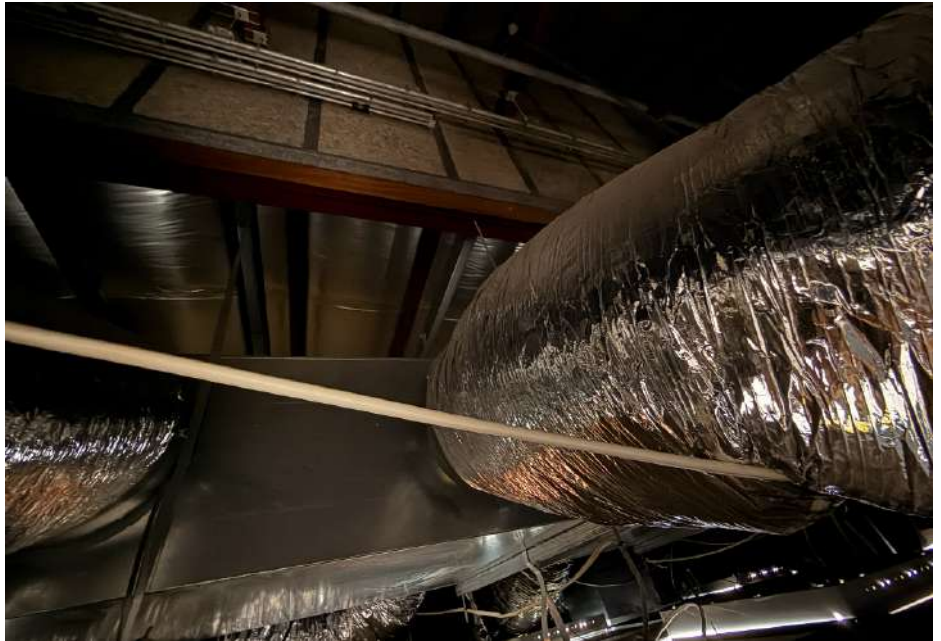
Figure 51 – Ceiling space of auditorium, showing all original ceiling timbers removed and filled with services
