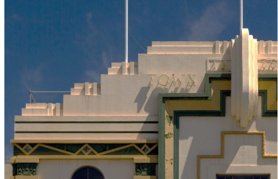
Port Road elevation parapet detail showing receding steps and rising dentils
