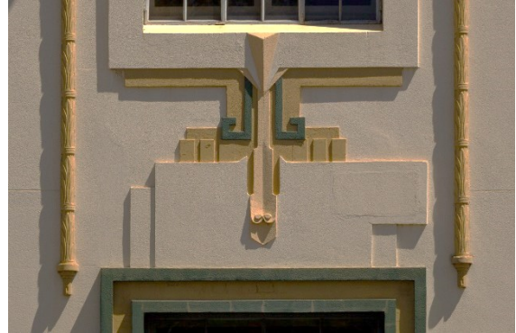
Decoration to Port Road elevation showing keystone, Greek key and fern motifs
