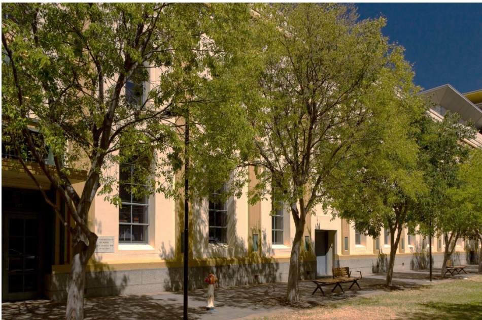
Milner Street elevation former Council Chambers and Institute Library (built in stages c.1860-1886, refaced 1936-1937)
