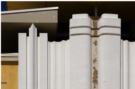
Detail of fin and trough features to former picture theatre entry
