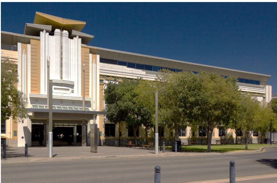
Milner Street elevation showing wall of picture theatre (built new 1936)
