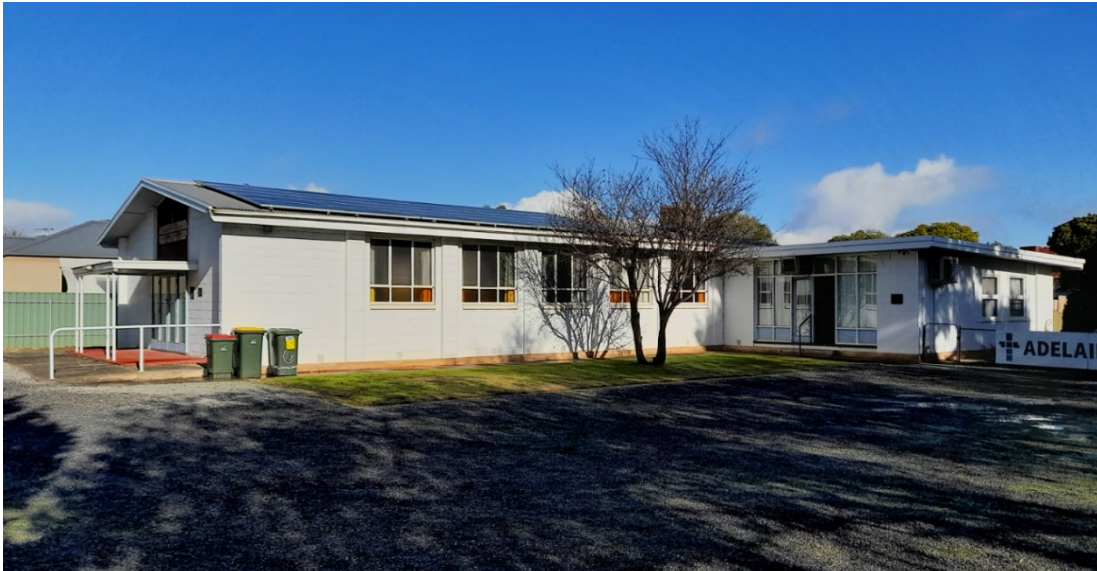
Jean Flynn Presbyterian Church, showing chapel (left) and hall (right).
