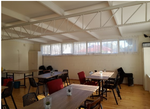
Interior of hall viewed from entrance.
