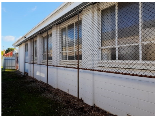
Freestanding chain-mesh fence structure protecting windows on southern side
