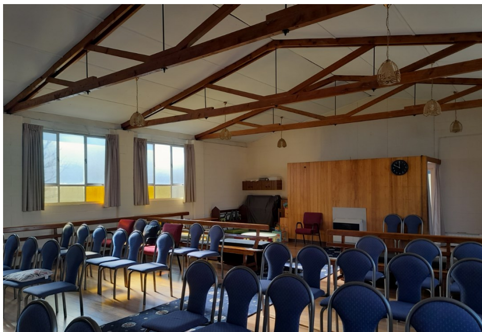
Interior of chapel, view towards entry
