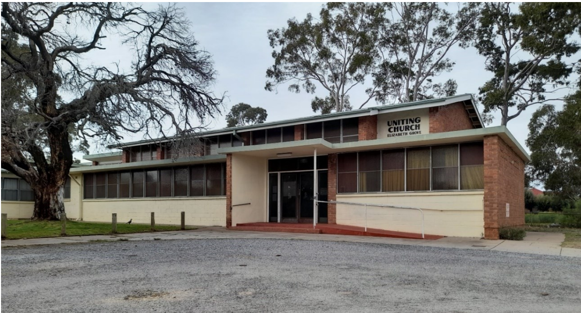
Former Elizabeth South Methodist Church Hall, northern side showing main entrance
