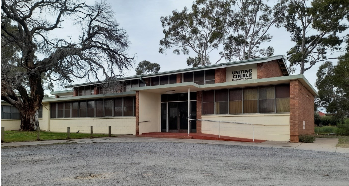
Former Elizabeth South Methodist Church Hall, northern side showing main entrance
