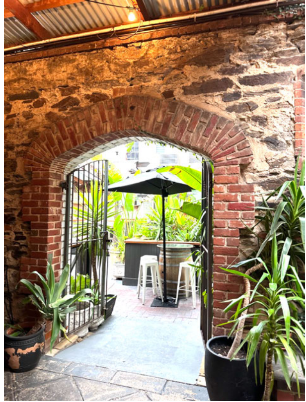
Figure 40: Western boundary wall of original stable, viewed from west (left) and one of two openings (right) which provided access between the stable yard to the private roadway along the western boundary.
