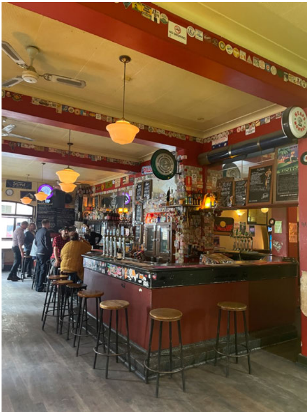
Figure 41: Original 1850s bar area (left) and 1920s dining room (right) indicating earlier wall locations in bulkheads and wall nibs
