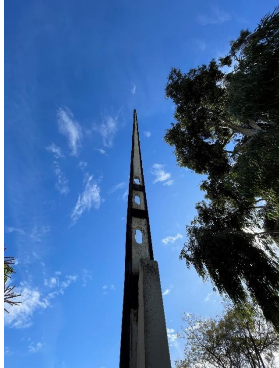
Rear of the 1924 Stobie pole showing tie bolts.
