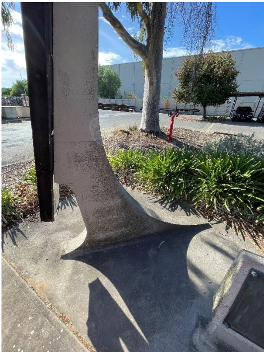
Original concrete base of the 1924 Stobie pole.
