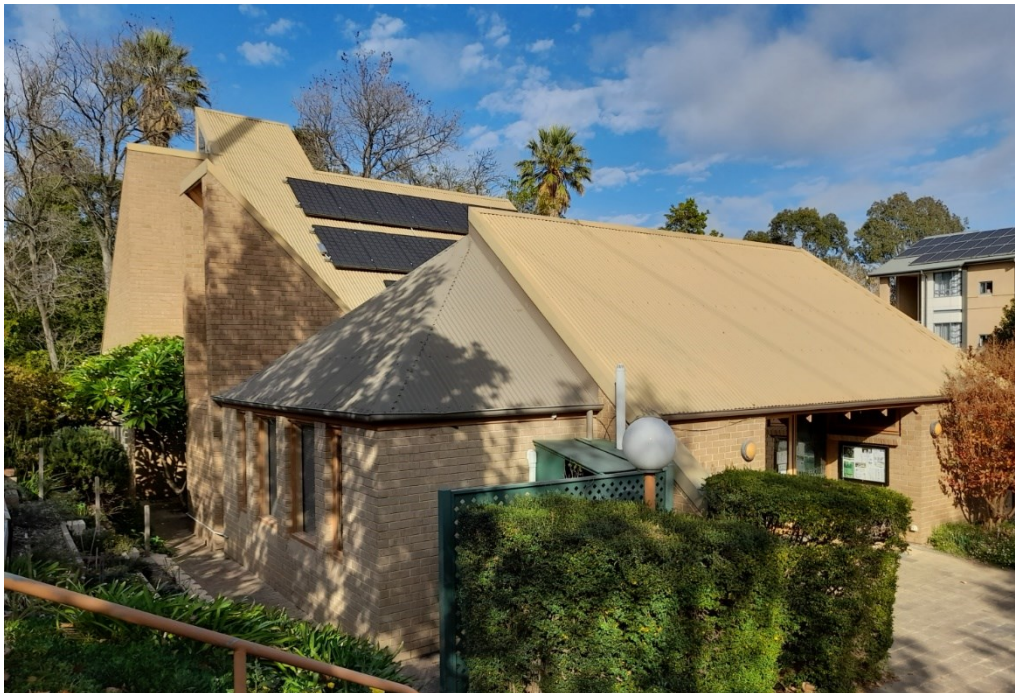
Christ Church Uniting (church), exterior showing entrance (on right), note hipped-roofed office extension on left
