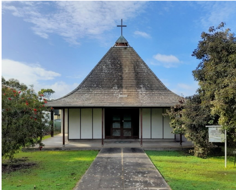
Former American River Methodist Church, northern elevation.
