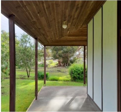
View under verandah showing lined soffit
