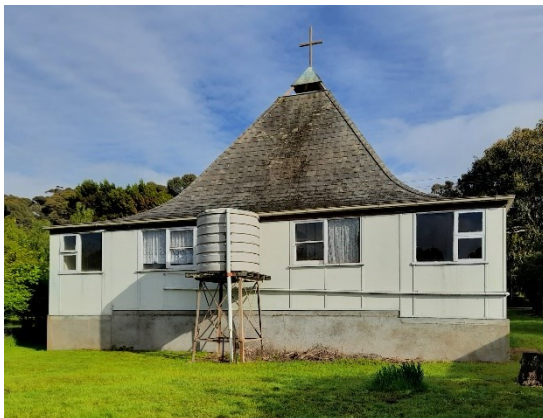
Southern elevation showing enclosed verandah
