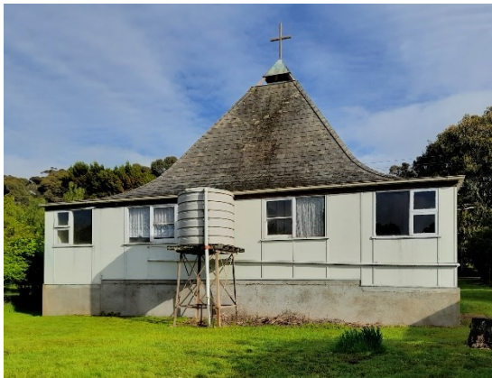
Southern elevation showing enclosed verandah
