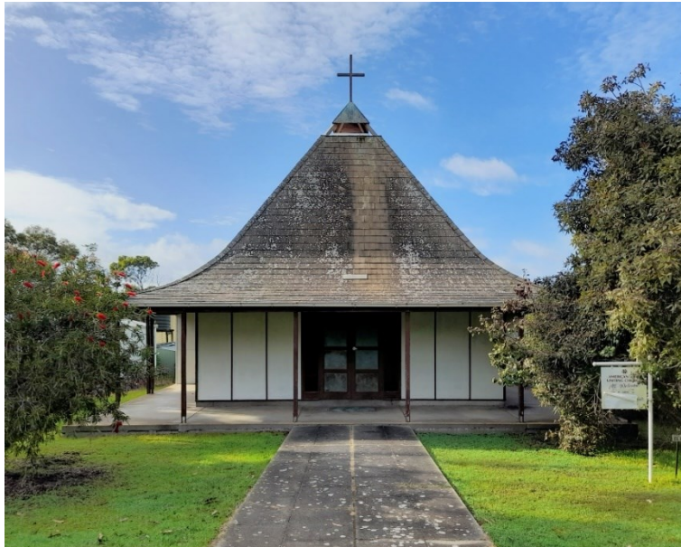
Former American River Methodist Church, northern elevation.
