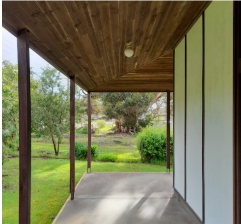
View under verandah showing lined soffit
