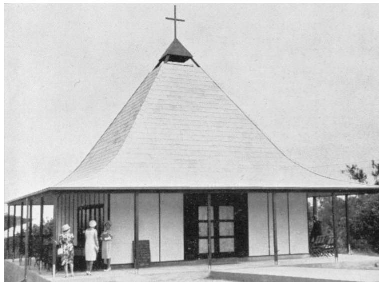
American River Methodist Church, pictured soon after completion, c.1966, note collapsible seating arranged under verandah to serve a holiday overflow congregation.
