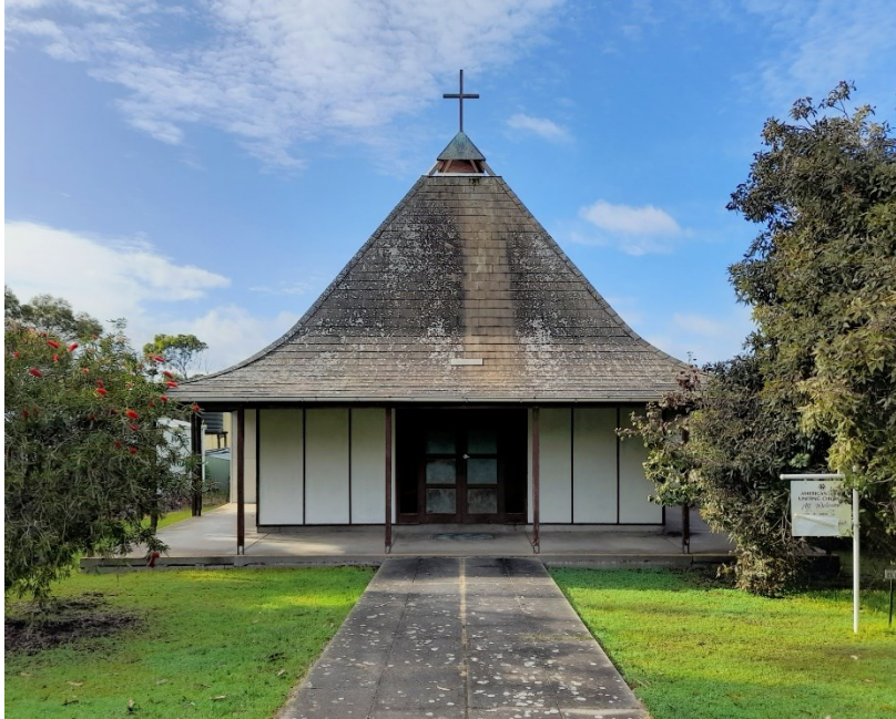
Former American River Methodist Church, northern elevation.
