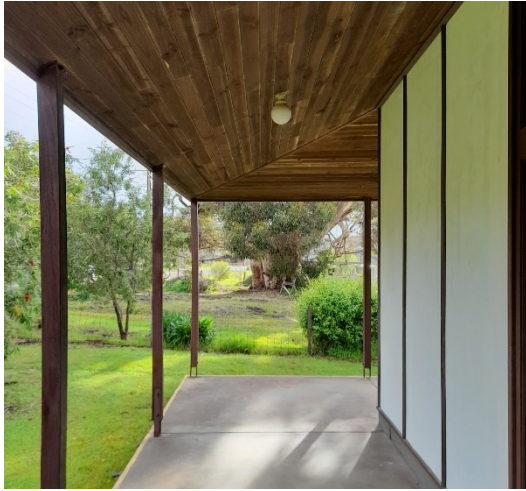
View under verandah showing lined soffit
