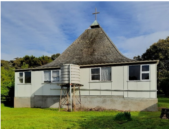
Southern elevation showing enclosed verandah
