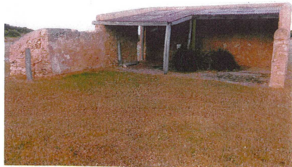
Historically inaccurate rebuild of northern wall - Business poorly taken on 1- 1995 Pas 1890s Dring
