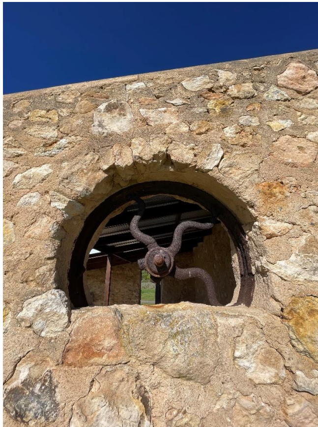
Semi-circular window with non-original iron insert on northern elevation of Dairy One.
