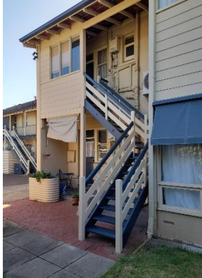
Typical rear staircase structure
