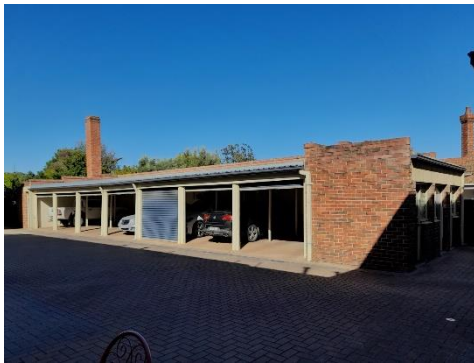
Laundry, garage and incinerator block, note chimney at eastern end
