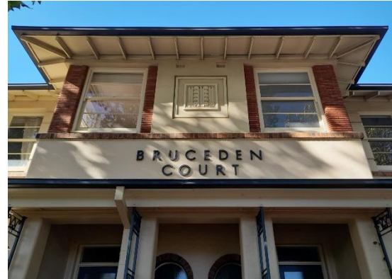
Detail of Cross Road elevation
