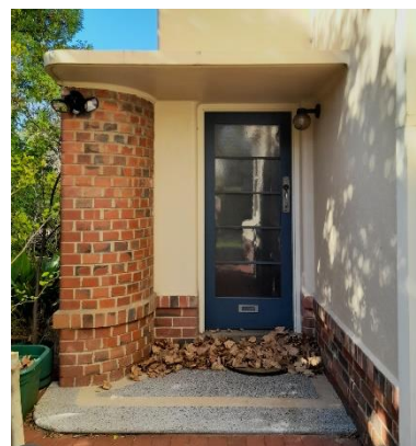
Entry with curved brick wing wall
