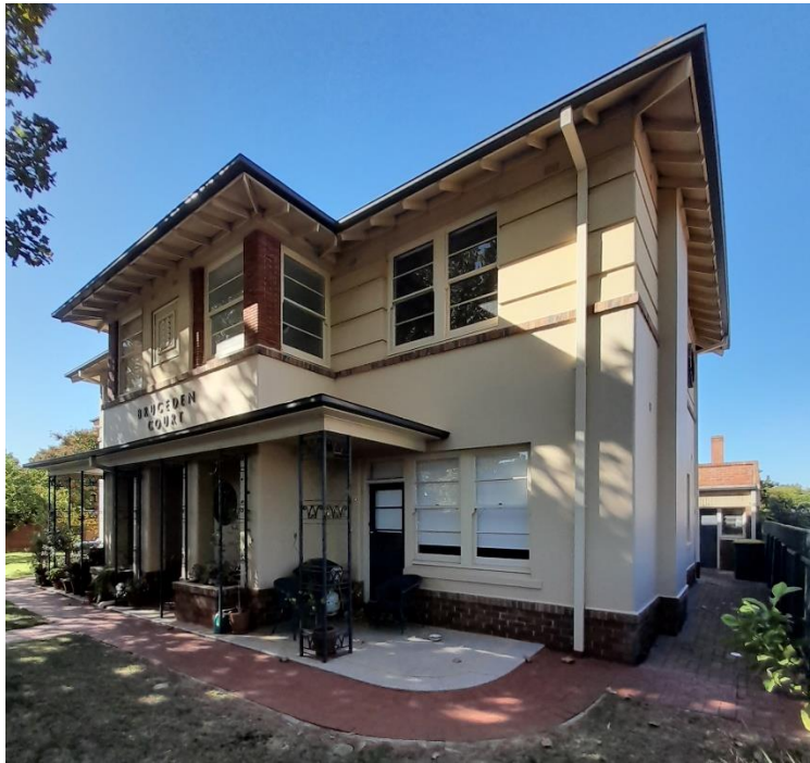
Bruceden Court, Cross Road elevation
