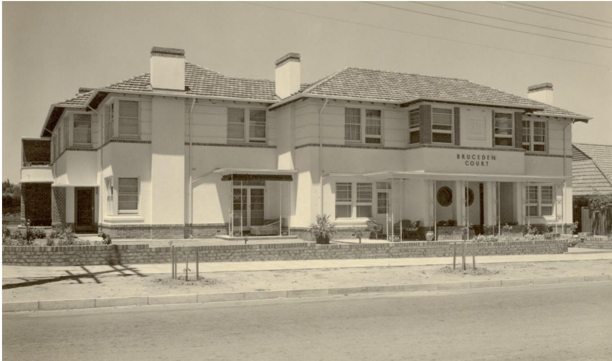
Bruceden Court (flats), c.1941, showing front elevation of duplex (two-storey) flats
