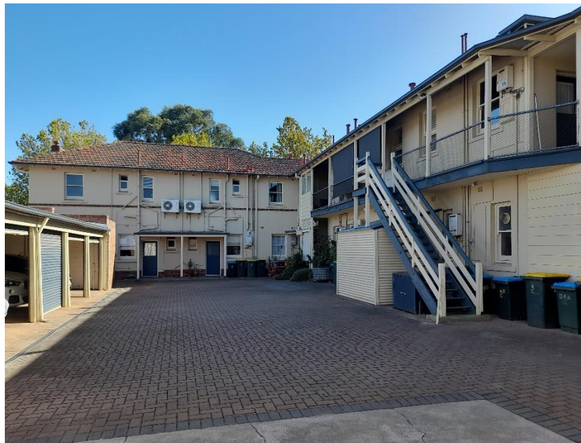
Rear elevations, with garage doors on left
