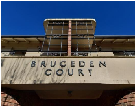
Balcony detail on Deepdene Avenue elevation
