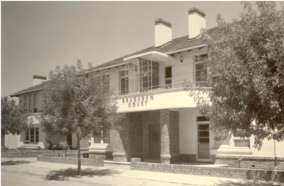
Bruceden Court (flats), c.1941, showing front elevation of simplex (single-storey) flats
