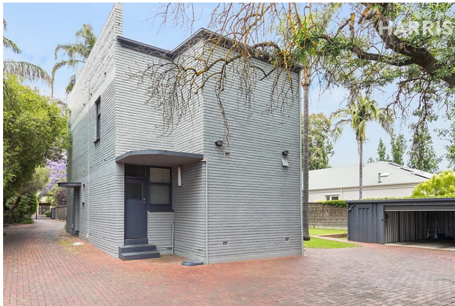
Rear view looking south-west
