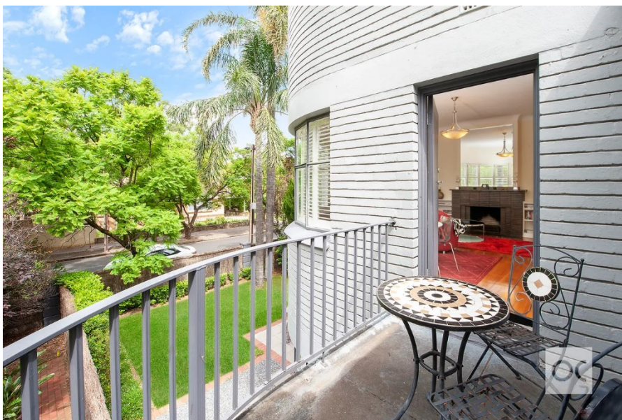
Upstairs balcony showing horizontal raked pointing
