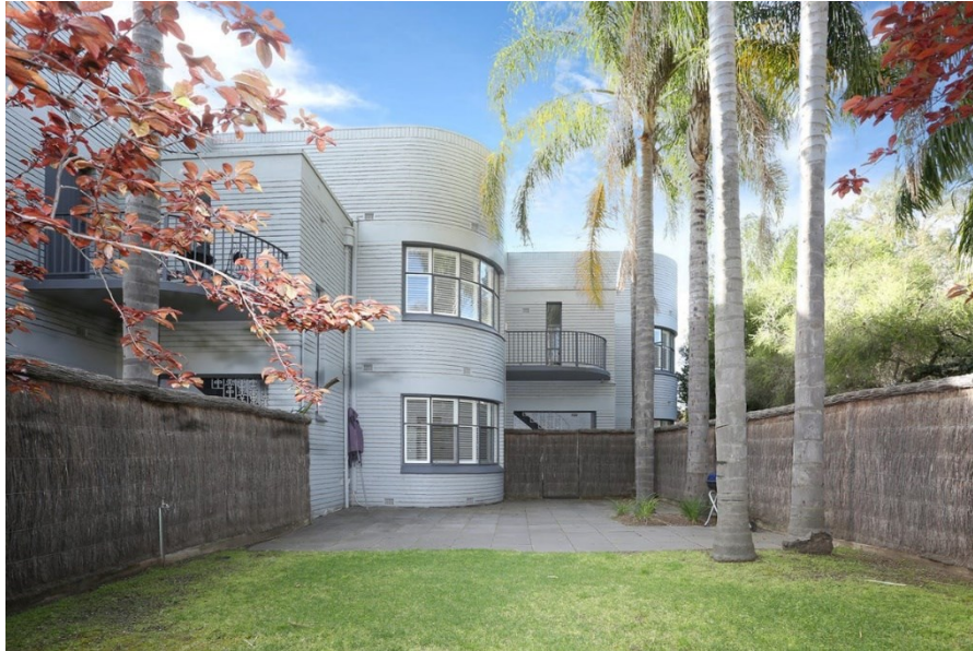
Front view looking north
