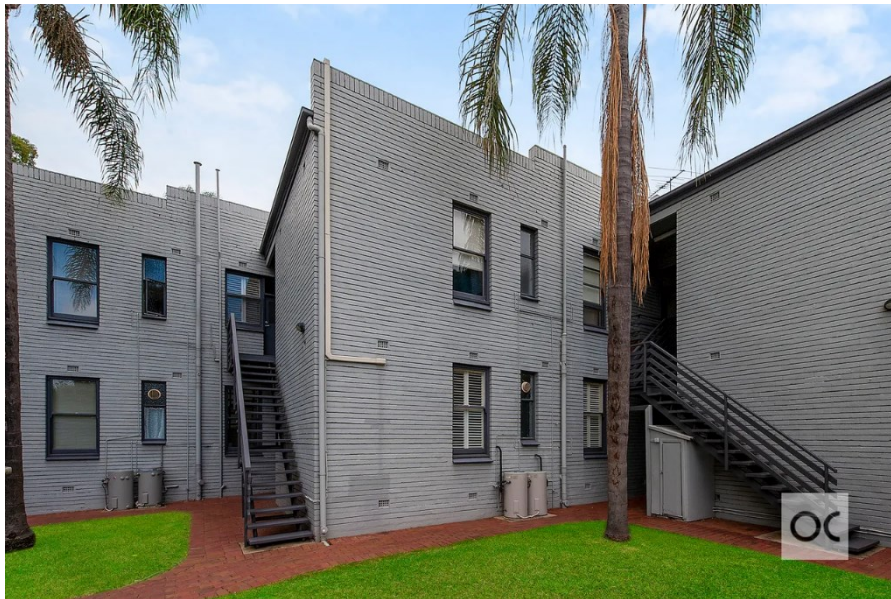
Rear view looking south-east
