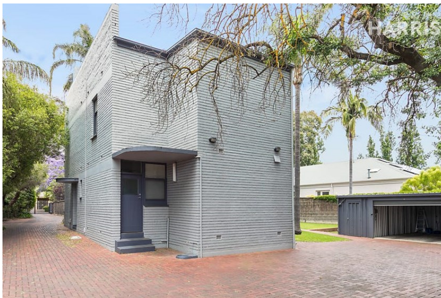
Rear view looking south-west
