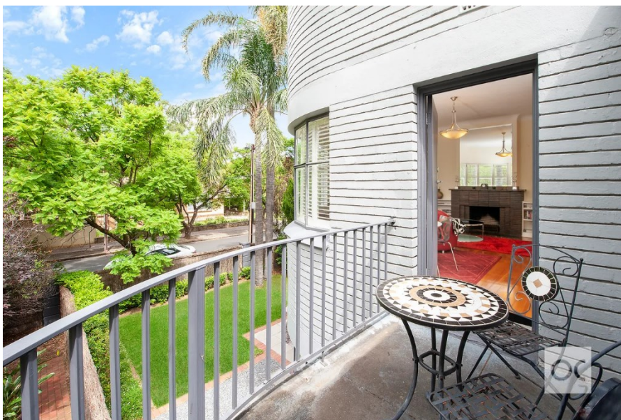
Upstairs balcony showing horizontal raked pointing
