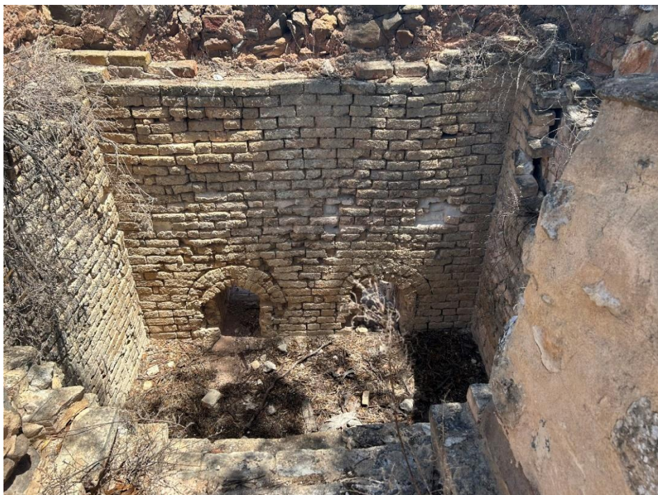
Interior of the western lime kiln. This kiln retains its double-layered fire brick lining.
