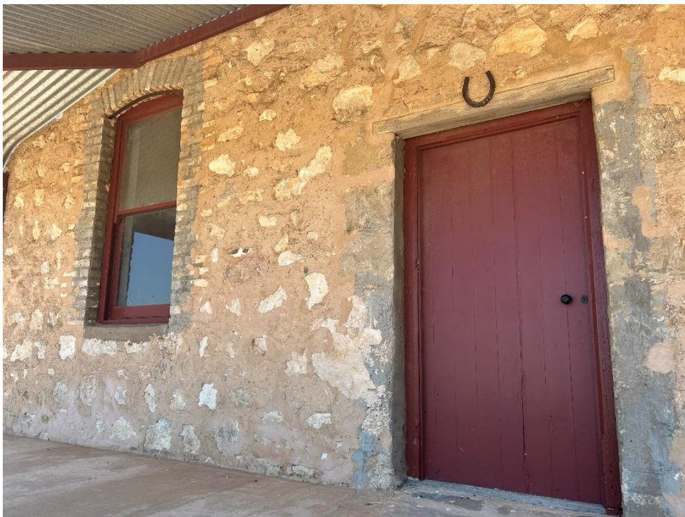
Door and window detail of the Bretag cottage, note the use of the firebricks from the kilns to window surrounds.
