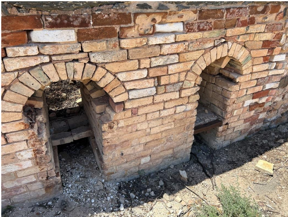
Lime kiln fire door archways.
