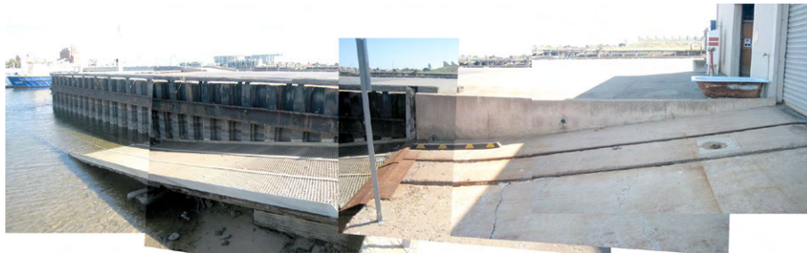
Figure 3.192 The slipway leading up to Shed 18. A timber ramp structure is visible below the metal grating. Image: Mulloway Studio
