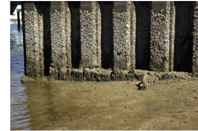
Figure 3.193 A timber structure is visible to the outside face of the existing steel sheet piling on the former salt company wharf. Photograph: James Bateman
