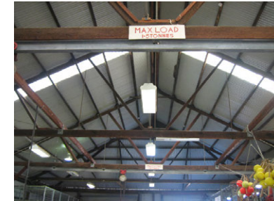
Figure 3.189 Timber roof structure of Shed 17 looking north. Some crane pulleys have been installed in the central shed area. Image: Mulloway Studio
