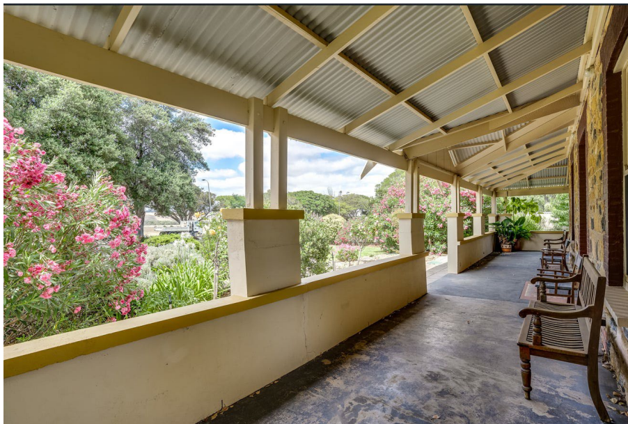
View of the verandah.
