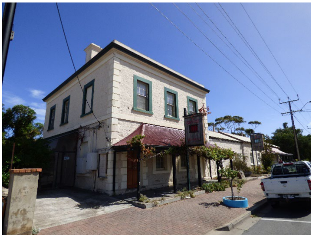
Former Normanville Police Station, Normanville, from 1855, (SHP 26470), 2017.
