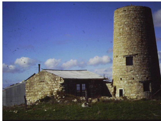
Former Currency Creek Mill, Currency Creek, 1855-1864 (SHP 10351), c.1980s.
