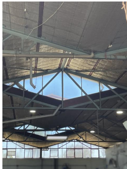
Roof trusses in factory forming rhomboid skylights.
