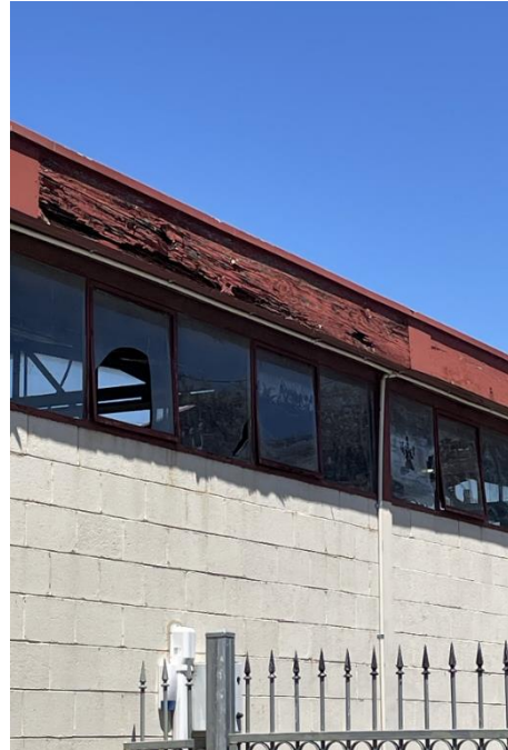
Indicative damage to facias (rot) and glass.
