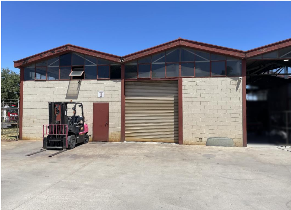
Section of the factory's northern (rear) elevation showing gable truss roof pattern. Note that the Besser blocks have not been painted.
