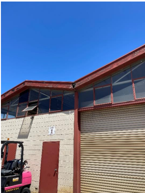
Indicative damage to fascias on northern elevation.
