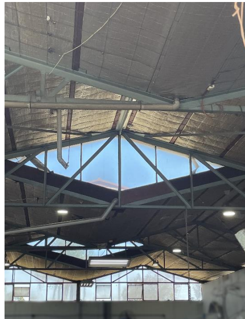
Roof trusses in factory forming rhomboid skylights.
