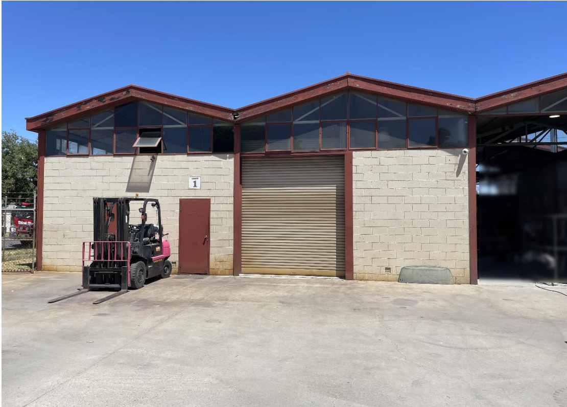
Section of the factory's northern (rear) elevation showing gable truss roof pattern. Note that the Besser blocks have not been painted.
