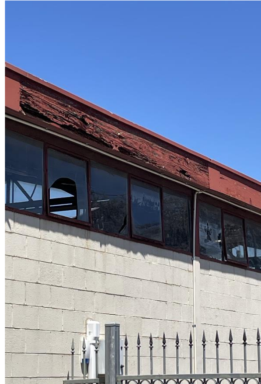
Indicative damage to fascias (rot) and glass.
