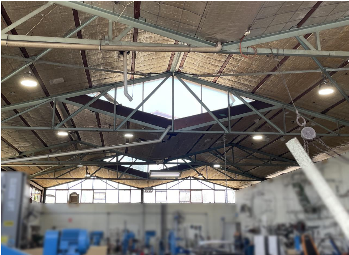
Interior view of factory showing steel trusses, rhomboid skylights, clerestory windows and insulation (Sisalation).
