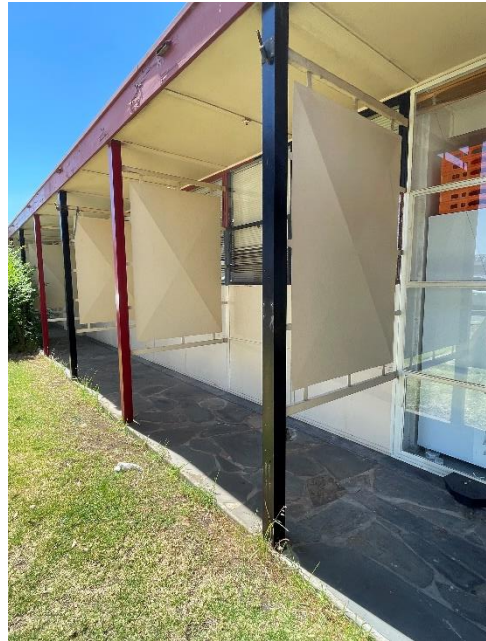
Eave at southern elevation with steel posts and fins.
