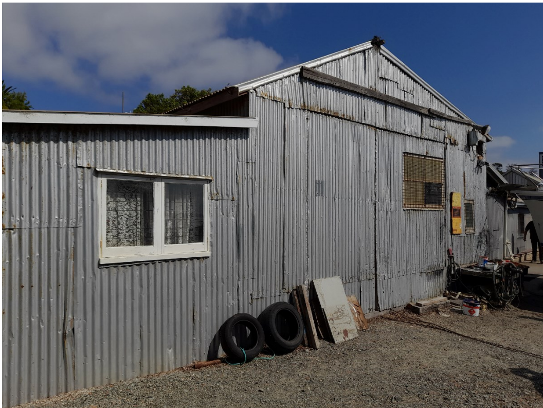
Former A. A. Stenross & Company Boatyard, showing front of workshop building.
