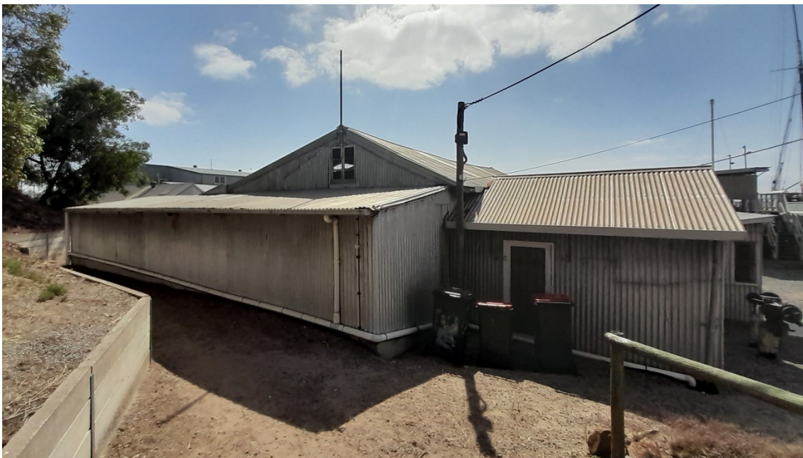
Rear view of workshop sheds.
