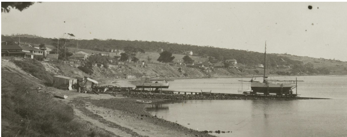
The Gulf Docking Company slip, adjacent to Tasman Terrace, while owned by A. A. Stenross & Co, with two vessels on the slip, c.1930
