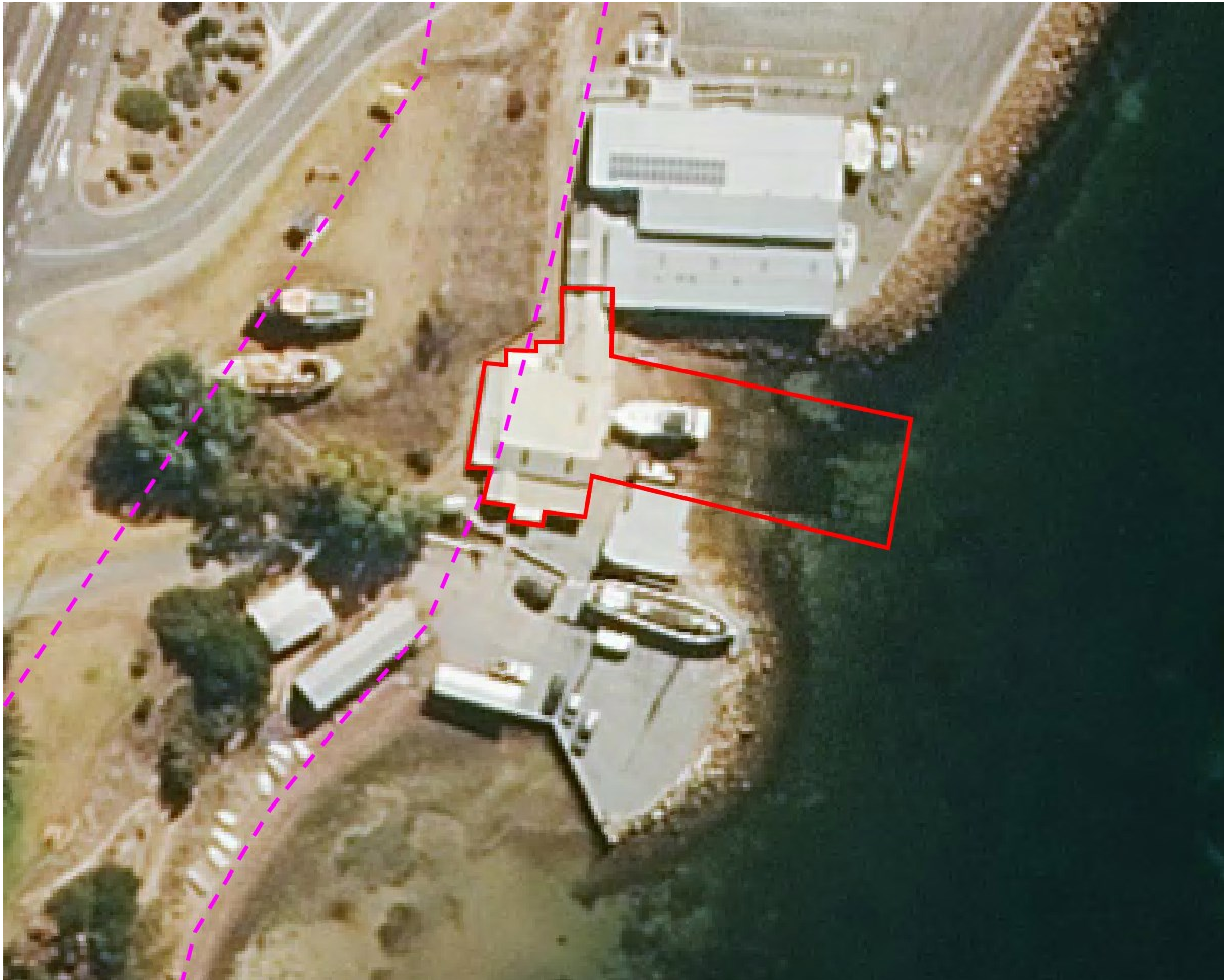
Former A. A. Stenross & Company Boatyard (detail)*
