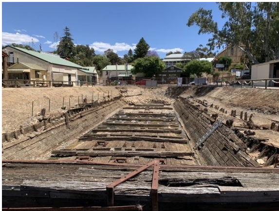
Former 'Randell' Dry Dock, 1873, Mannum (SHP 10282)
