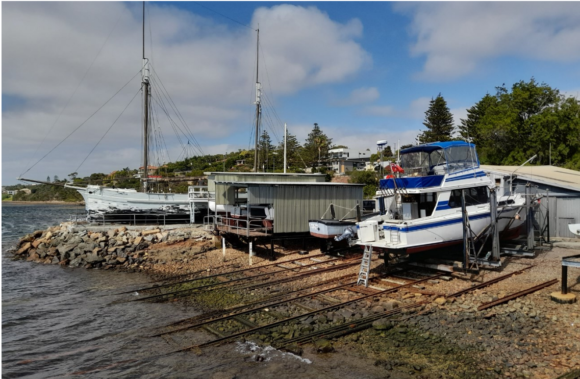
Slipways with workshop sheds in right background.
