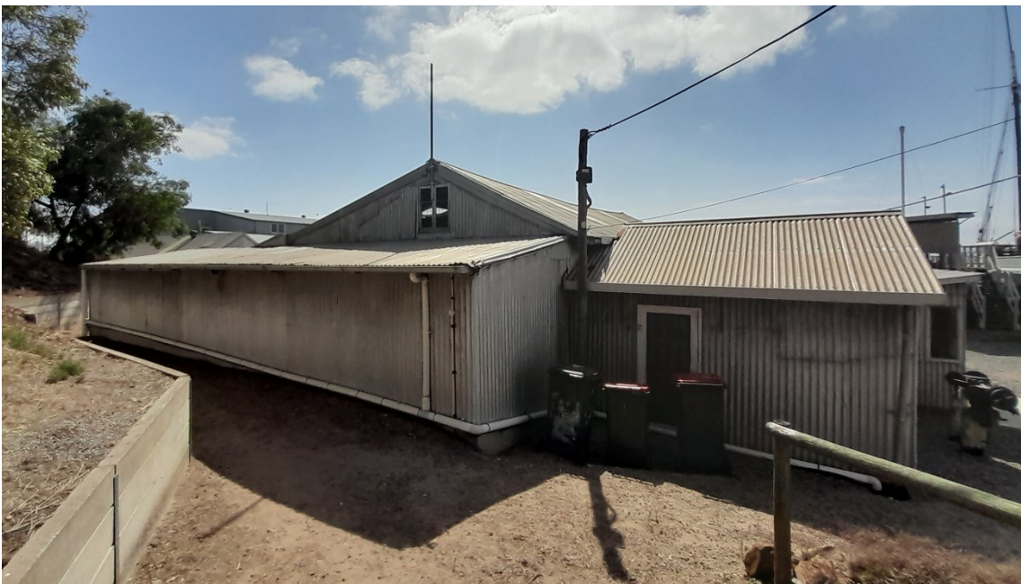
Rear view of workshop sheds.
