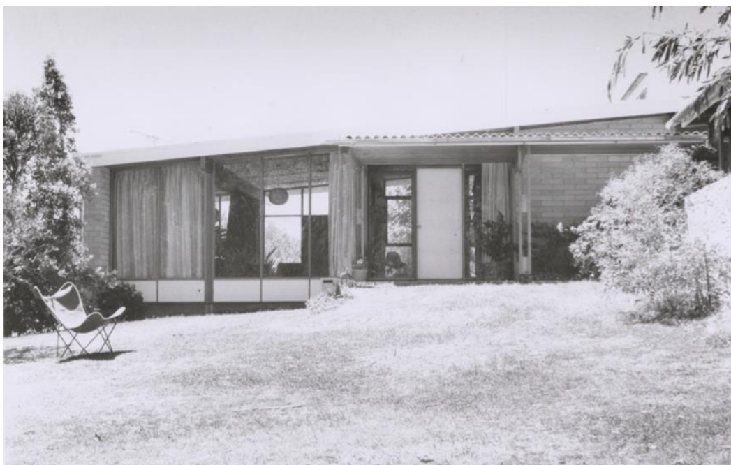
Southern (front) elevation of the Graham and Barbara Dickson House, showing living room (left), front door with timber covered walkway and carport just visible to the right. Note the expansive use of glass with awning windows. The asbestos tiles are also evident on the covered walkway to front door and have since been replaced.
