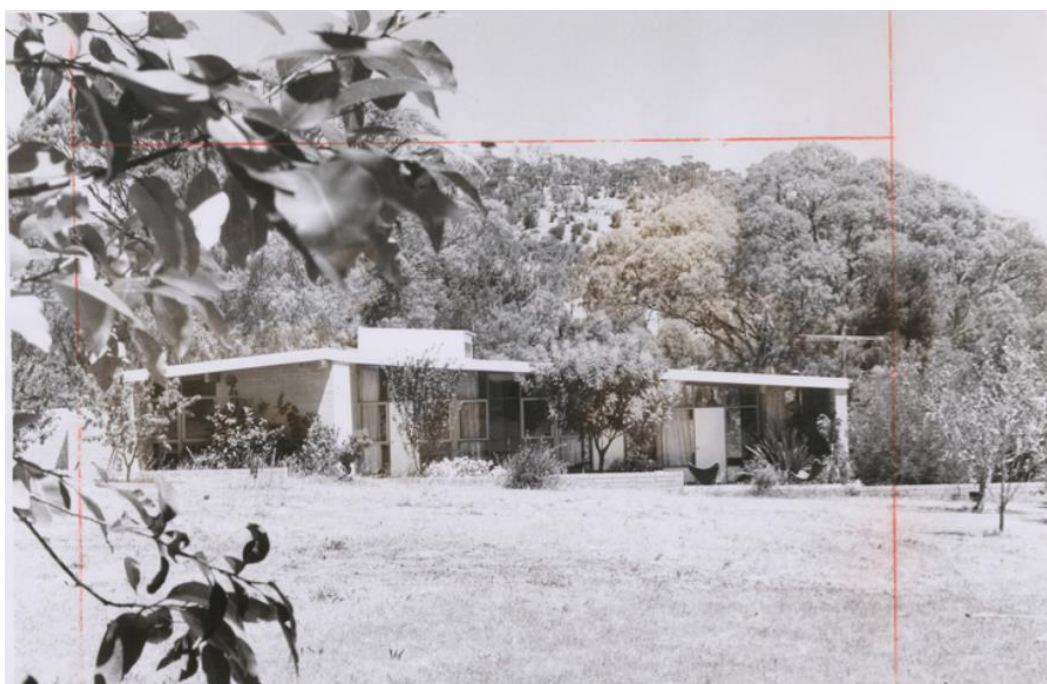
View of northern (rear) elevation showing the roof line matched to the slope of the site and the three stepped levels comprising bedrooms and bathroom (left) kitchen, dining and laundry (middle) and living (right). Note the expansive use of glass to provide an outlook over the garden. The new master bedroom and ensuite was added shortly after the image was taken.
