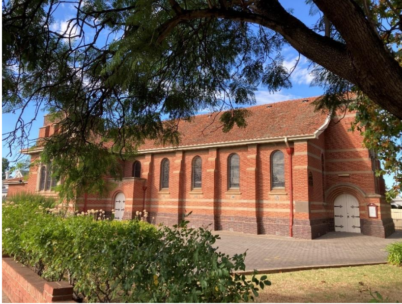
View of north-eastern elevation. Note the buttresses and round-headed openings.
