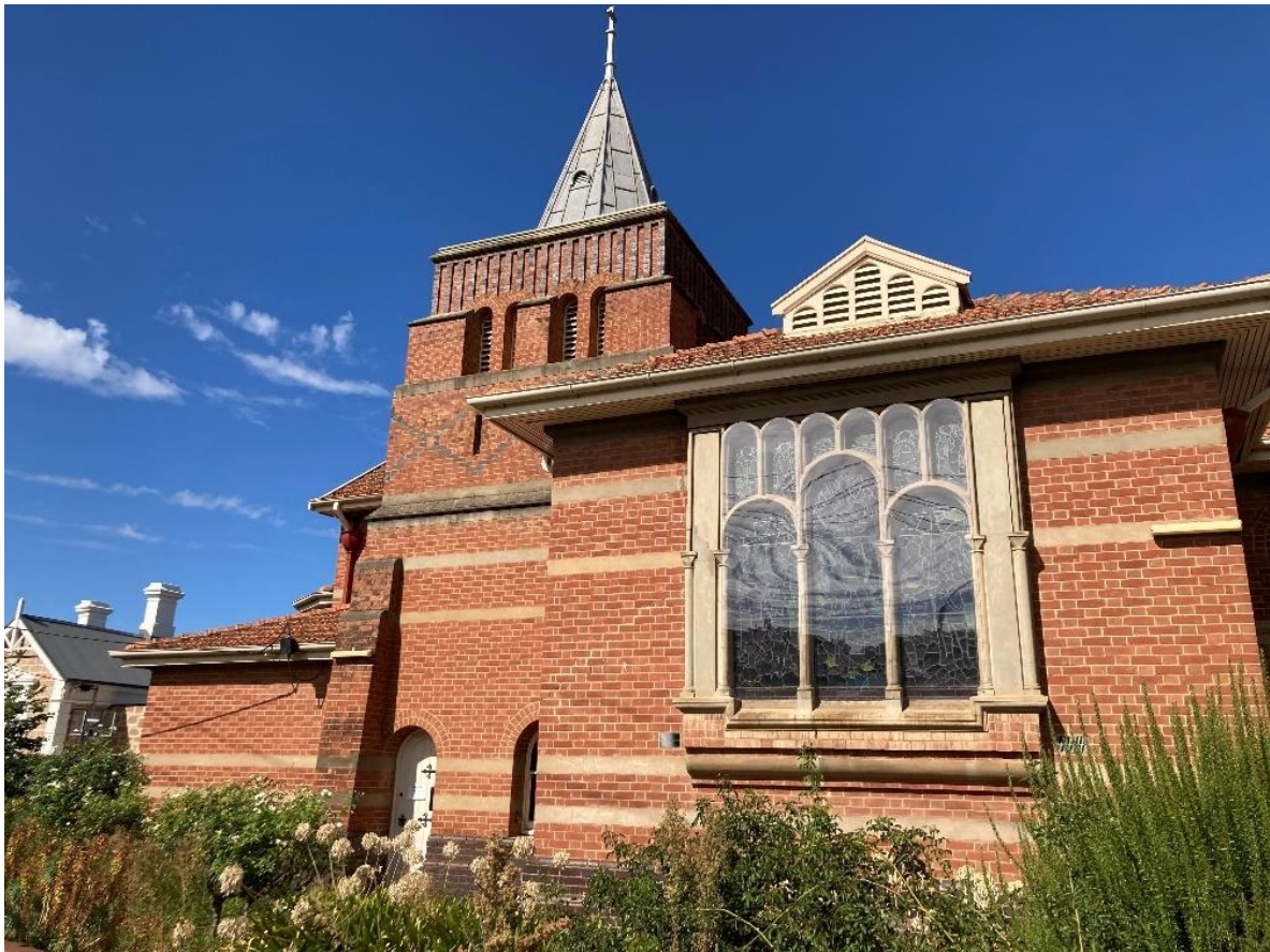
View of detail to transept windows. Also note the relief, vitrified-brick decoration to top of the tower and diaper work below round-headed vents.
