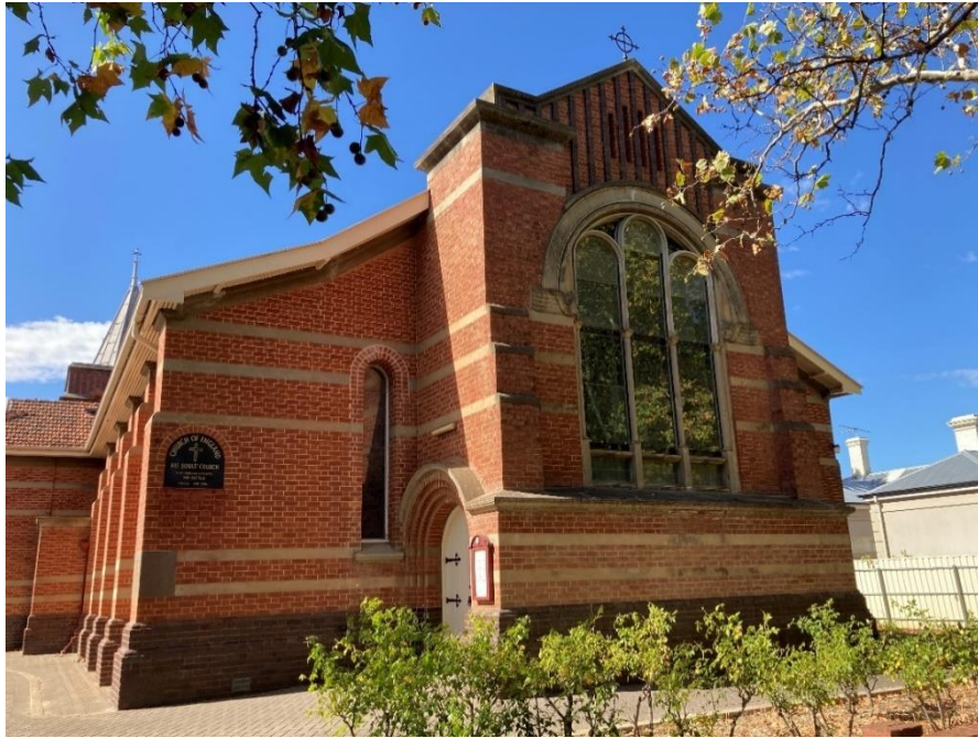
View showing the east window and detailing to narthex. Note stepped surrounds to doors, cement bands, and vitrified brick to gable.
