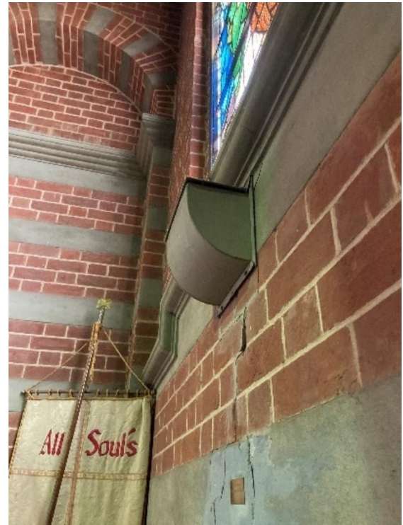
Detail showing the ventilation.
