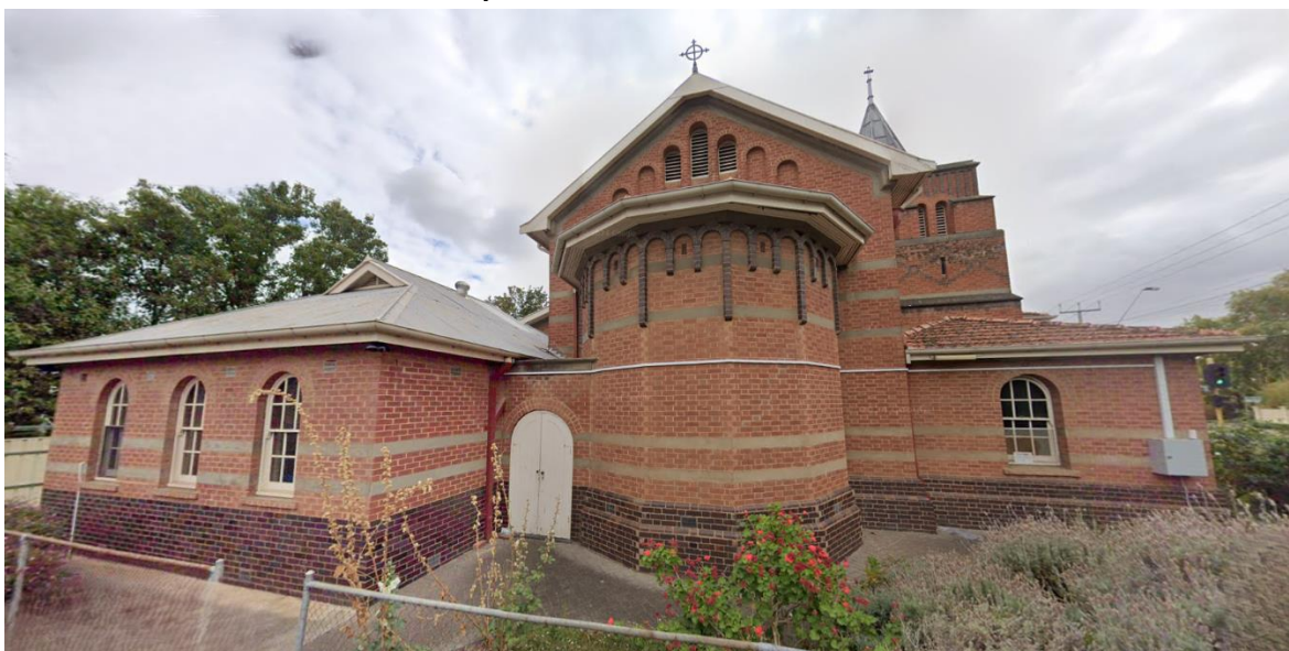
View of apse (middle), with blind round-headed and ventilation openings above, Kay Hall (left) and vestry (right). Note vitrified-brick plinth, relief details to apse, diaper-work to tower and use of similar detailing and materials in simplified form to kay Hall.
