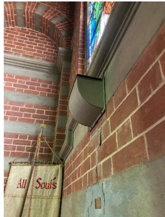
Detail showing the ventilation.
