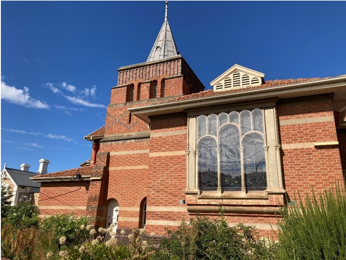
View of detail to transept windows. Also note the relief, vitrified-brick decoration to top of the tower and diaper work below round-headed vents.
