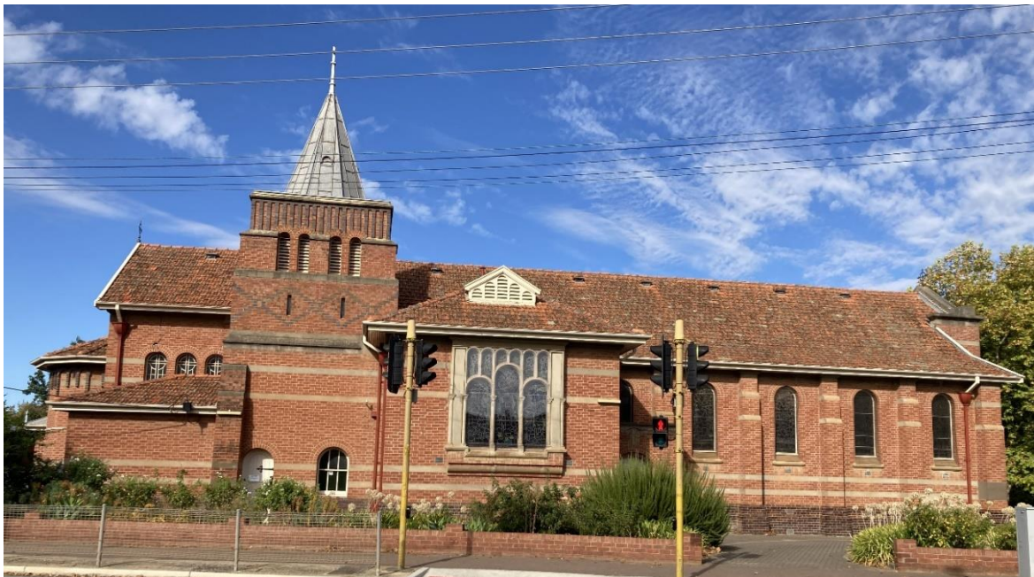
All Souls' Anglican Church, St Peters view of the north-eastern elevation.
