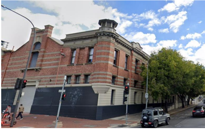
Adelaide Electric Supply Co. Power Station (now Tandanya), Adelaide, (SHP 10984), (1901).
