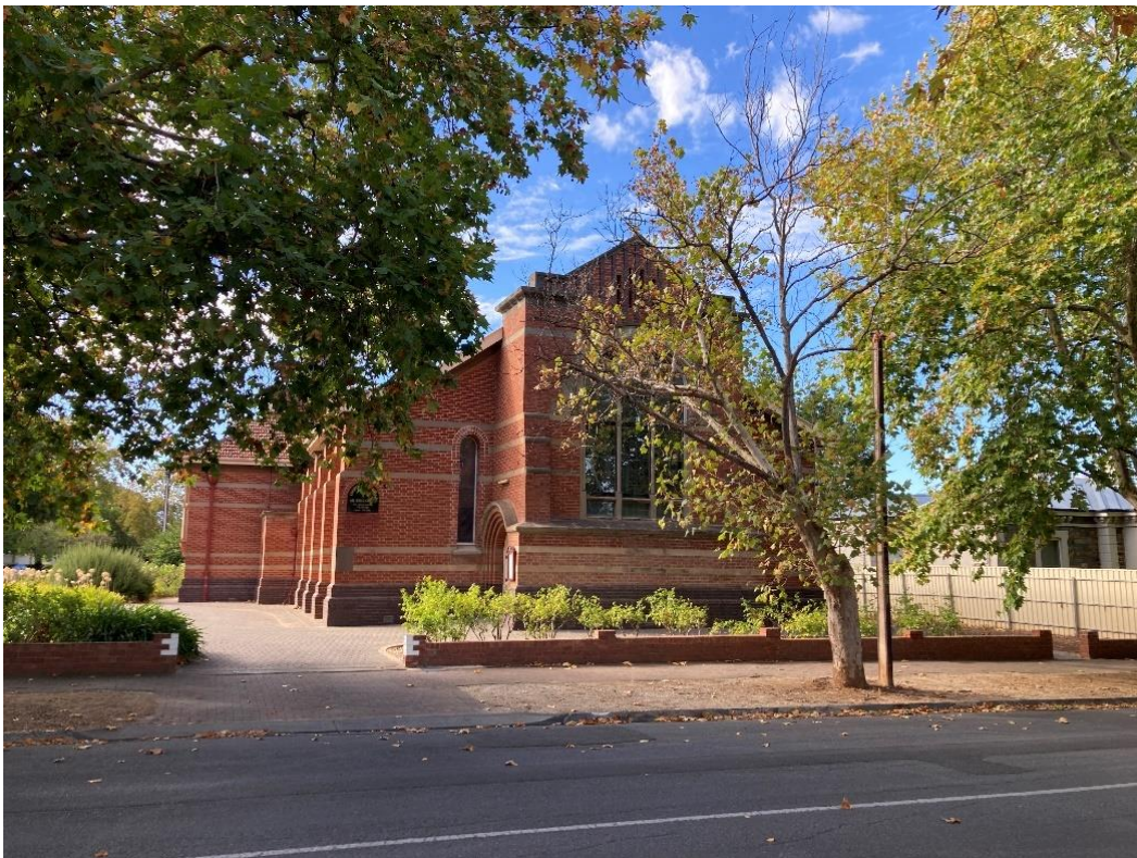
View of narthex. Note the garden wall.
