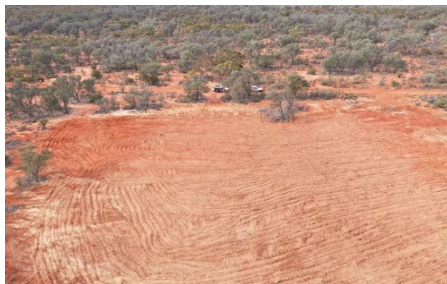
Photo 223. Little Oak Dam bulldozed flat; May 2019.
