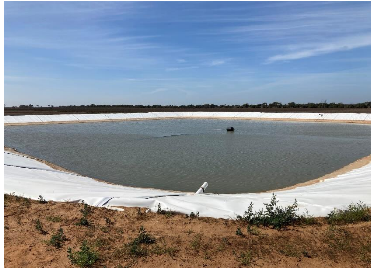
Photo 8. New storage dam installed as part of the Water Efficiency Program.
