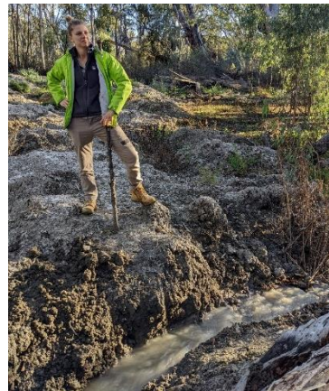
Photo 16. Wiela Bank breaching.
