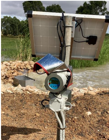
Photo 7. New water metering telemetry installed as part of the Water Efficiency Program.
