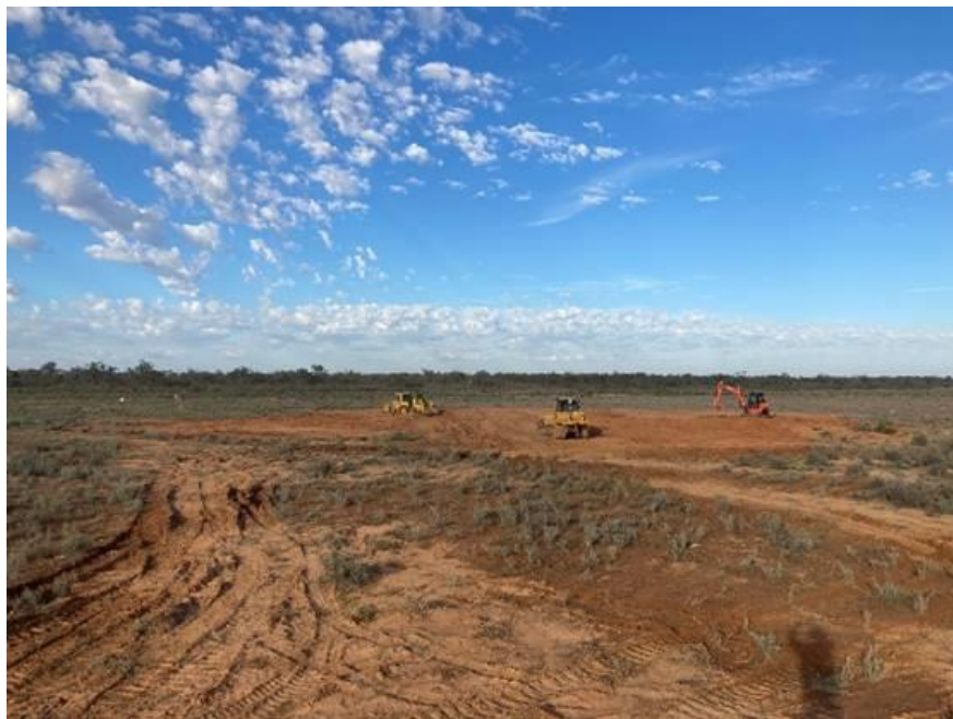
Photo 17. Dam decommissioning in process
