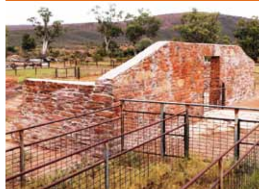
A stone wall restored by Mitsubishi 4WD Club volunteers on Moolooloo Station
