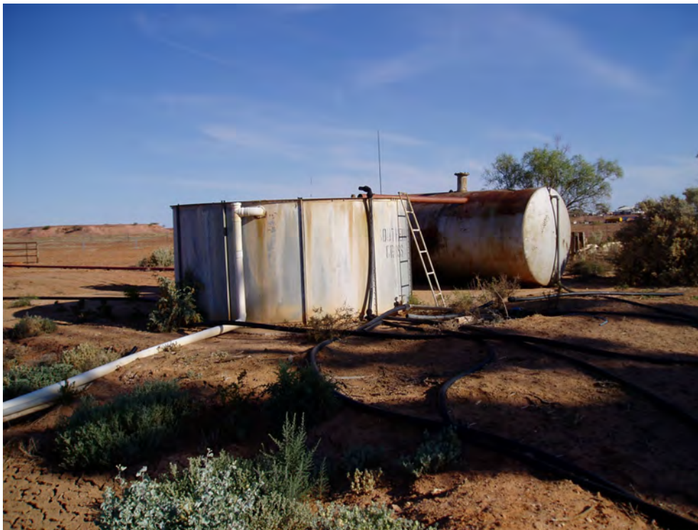
Figure 59 The balancing storage tanks at Murnpeowie, which overflow into the bore-fed wetland, 2004
