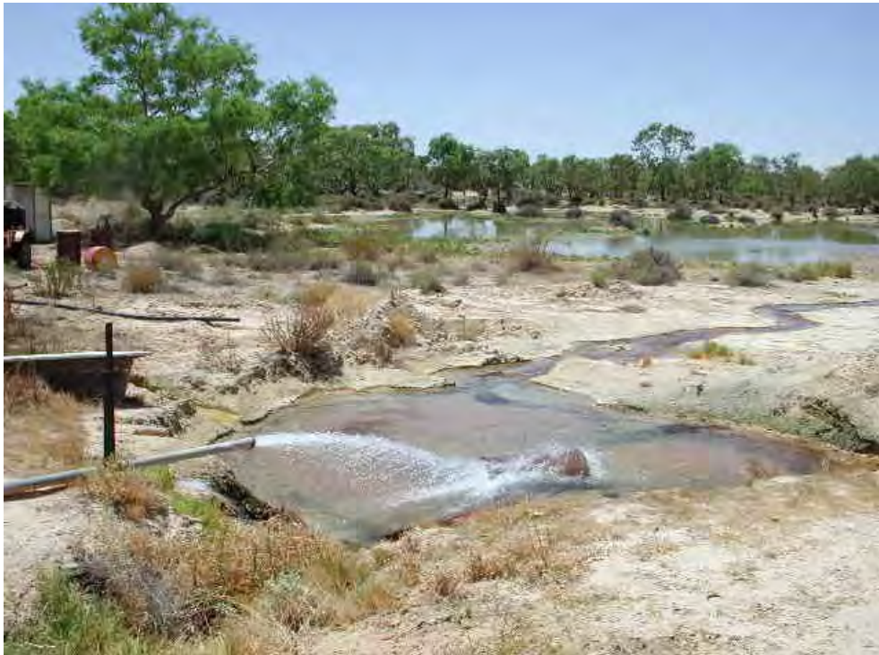
Figure 53 Current inlet pipe from the Lycium 1 bore into the Cooper Creek, February 2004
