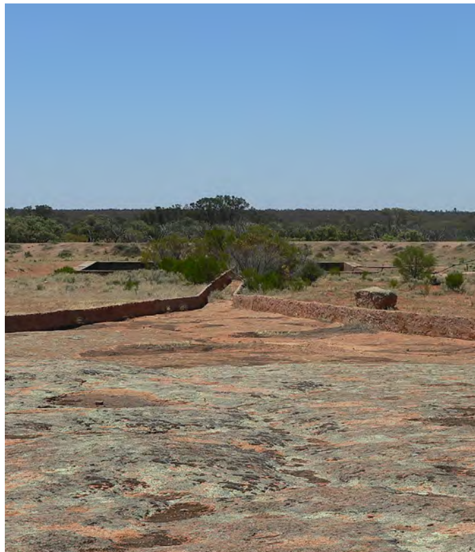
Figure 3.2 A granite pavement on Lake Everard Station in the Gawler Ranges that has had a stone wall cemented around its base to feed a water collection point (M. White, 2005)
