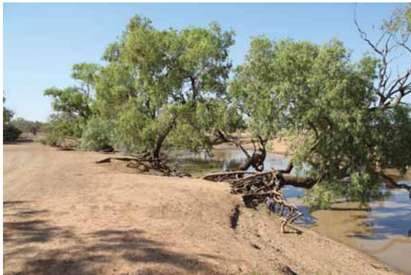
Figure 30. Stream bank erosion around camping activity site
