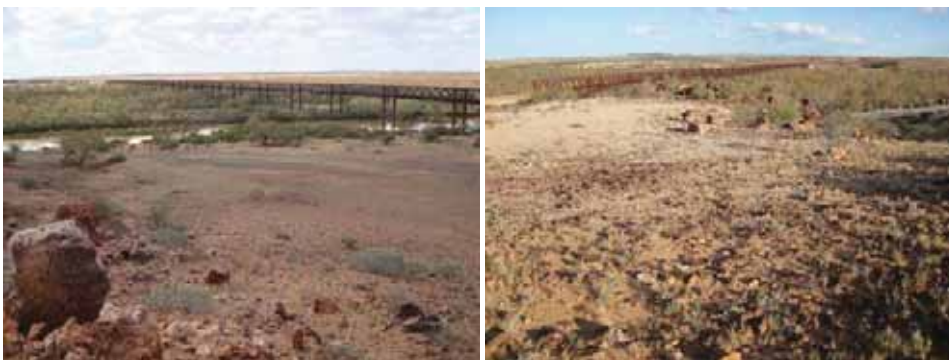
Figure 6.7.11 West Algebuckina south view over bridge toward west waterhole, West Algebuckina north view and East Algebuckina. Image: G Lee April 2010
