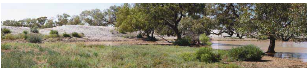
Figure 6.12.9 Dam limestone wall construction generally devoid of mature vegetation, a flat riparian treed zone with low samphire shrubland and grass understorey. Image: B Madill April 2010
