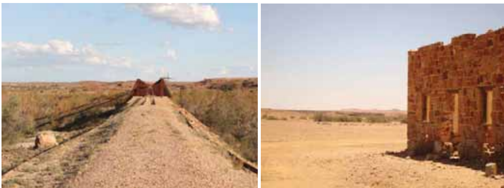
Figure 6.5.9 Algebuckina Bridge looking south, typical view looking southwest with fettler's cottage in foreground and the bridge beyond. Image: G Lee November 2009, April 2010
