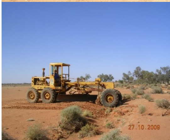
Reid's Paddock - Installing check banks below top contour bank and a gully head being addressed
