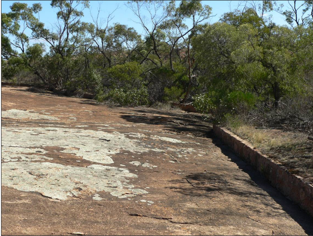
Figure 4. An example of a stone wall built around the base of a granite outcrop at Mt Wudinna on the Eyre Peninsula to capture rainfall run-off.
