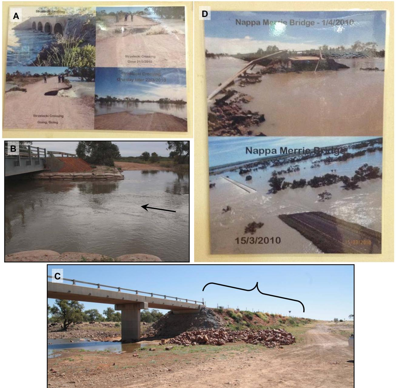
**Fig. 41. Increased stream power caused by poorly-designed road crossings.**
