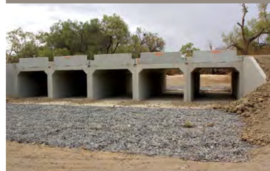
The new crossings will assist water and fish flow more easily through the Cooper
