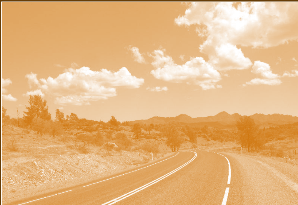
Work in progress on the Blinman - Wilpena Road (top), and the road newly sealed and line-marked.
