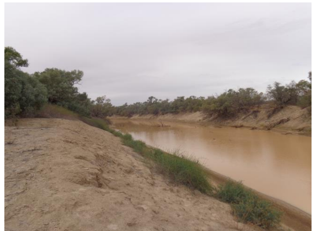
Diamantina River channelised section – steep banks
