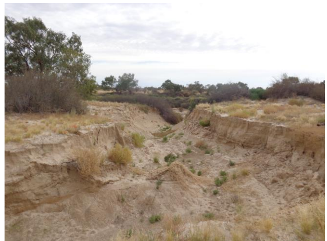
Increased erosion gullying 2016
