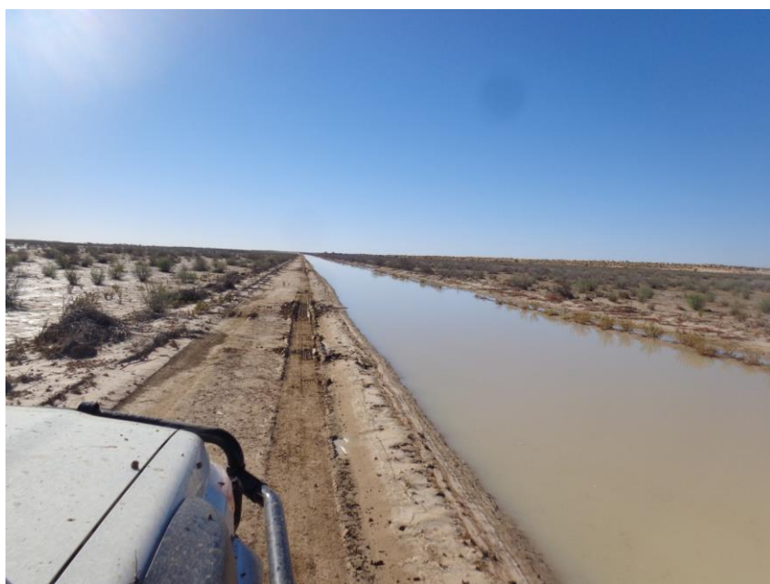
Figure 6 Inside Track – a surface water flow diversion forming a depression channel dewatering the surrounding landscape
