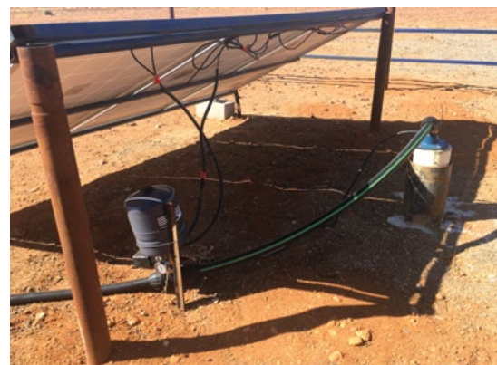
Installation of water-tight distribution to eliminate wasted flow at Elizabeth's Bore at Mount Barry
