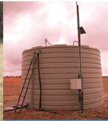
FIGURE 17 Closed water delivery systems ensure that water for stock is captured and delivered to stock through piped systems with tanks, float valves and troughs. (Photos: L Brake)
