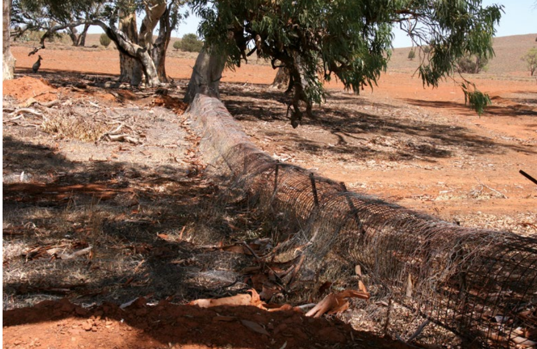
Debris traps constructed from mesh (above) and old fence material (below). Leaves and sticks have collected above the cylindrical barrier. Widening the breadth of the flow through the barrier has levelled out the watercourse downstream, which previously was a series of small ruts and channels.
