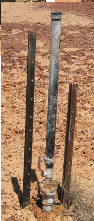
Air relief valves (ARVs) should ideally be installed at the top of each rise in the pipeline to release air from a pressurised pipeline during filling operations, and also to allow air to enter if the pipeline empties for any reason.
