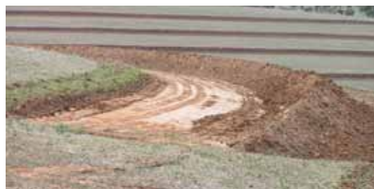
Above: Contour banks slow and move water safely across slopes.
