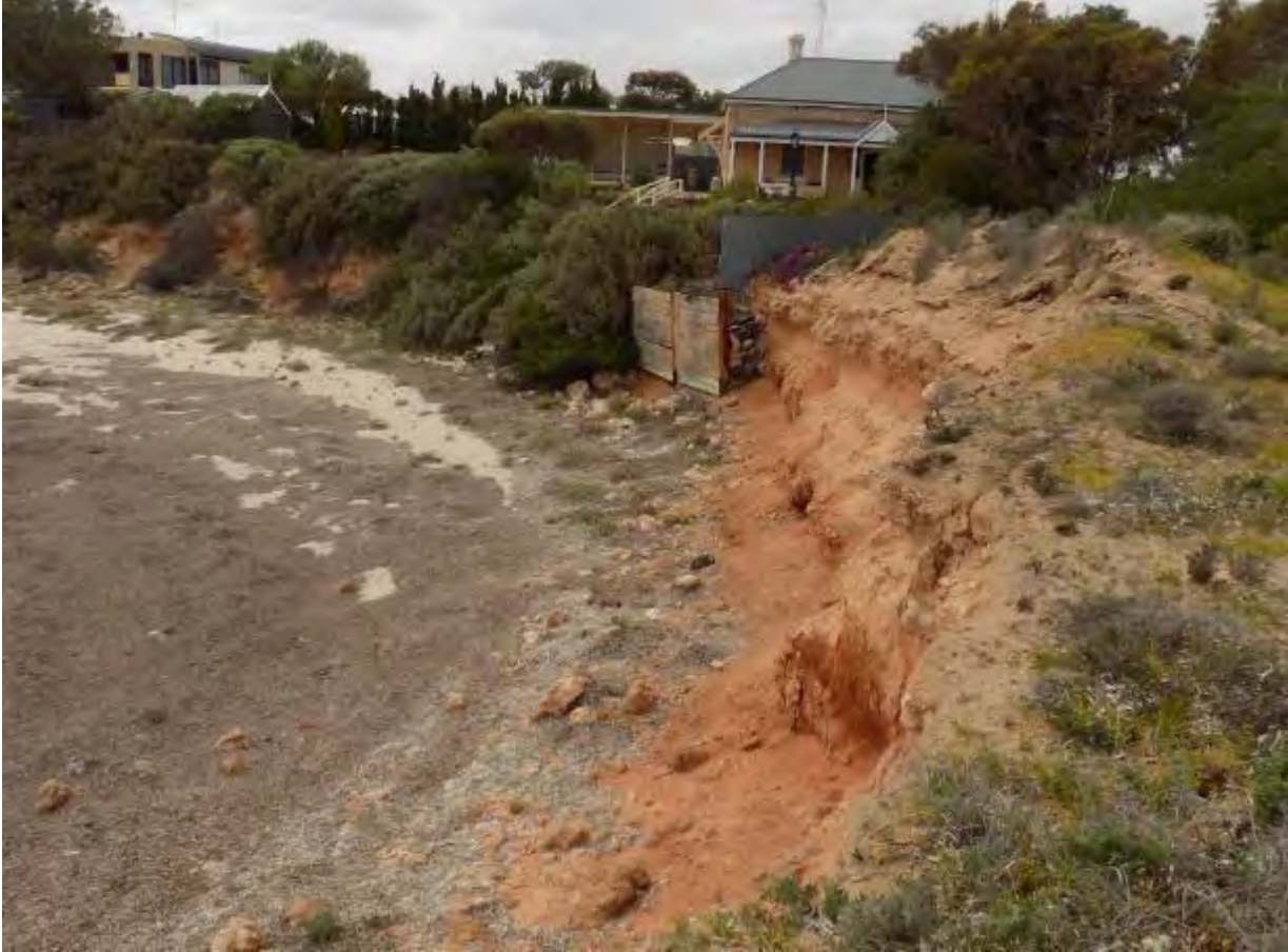
Photo: Low cliffs eroding at Moonta Bay forcing residents to reinforce fencing
