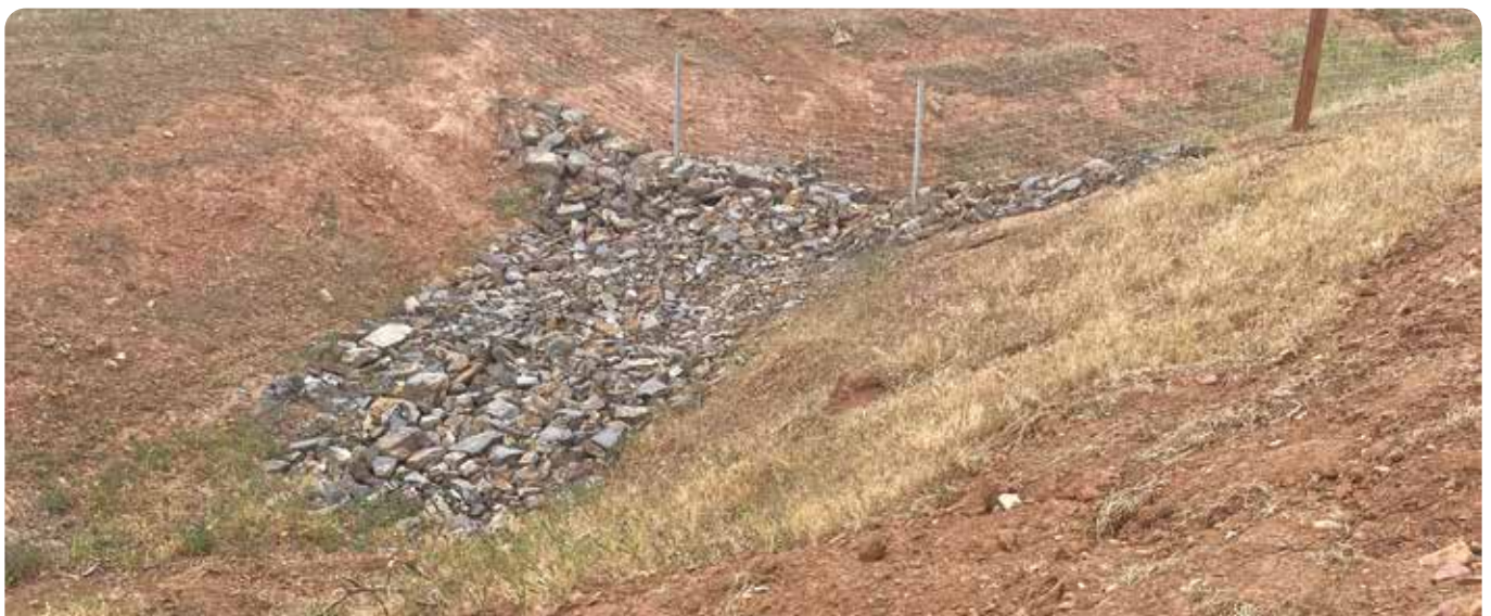
Stone fortification slowing water inflow at the inlet area.
