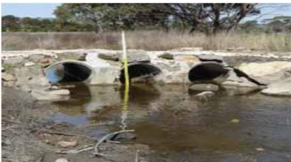
An example of a well-constructed crossing with adequate culvert sizing to allow fish passage and accommodate normal flows.
