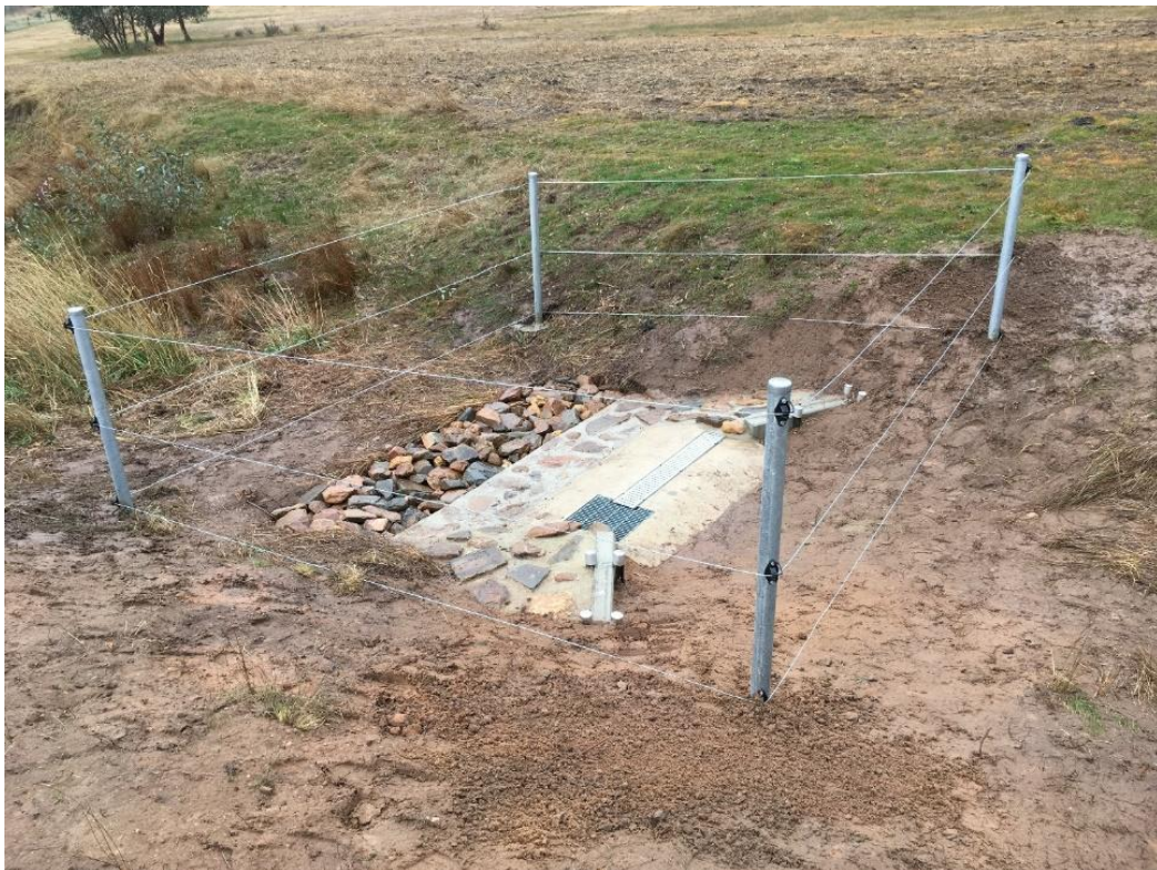
Figure 4: A typical low flow device. During periods of low flow, the device diverts water around the dam. During medium and high flows, water flows over the device and into the dam. Within the device is a regulator which limits the rate of flow that is diverted around the dam.
