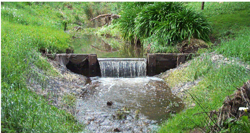
Figure 10: Timber weir, example of a structure
